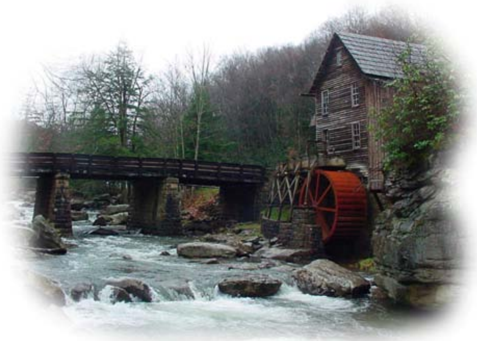
Figure 1—A stress-laminated road bridge constructed with creosote-treated wood near the Glade Creek Grist Mill in Babcock State Park, WV.
