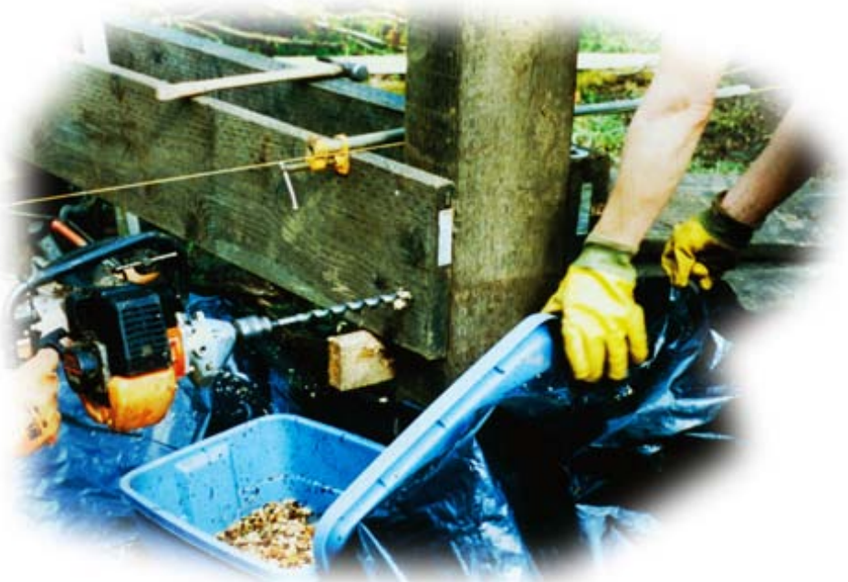
Figure 9—A tub can be used to collect sawdust when drilling preservative-treated wood. Collecting debris during construction helps to minimize environmental impacts.
